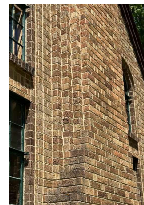
Stepped masonry chimney
