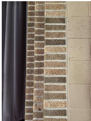
Stepped masonry proscenium
