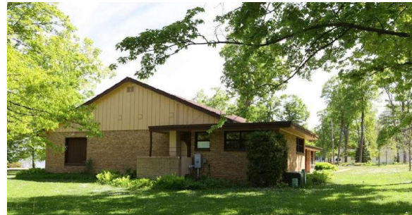
Rear Elevation Landscape does not screen views of utility infrastructure.
